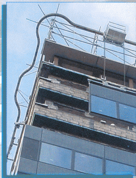
Monorail — on the left side the section, where it “doubles” the quick lift.
