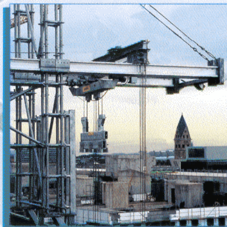
Outrigger with suspension points for a platform and spreader bar for lifting the façade elements
