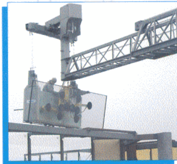
The jib section of the BMU with operatives in the cradle and a panel suspended from the material hoist and held by a vacuum lifter.
