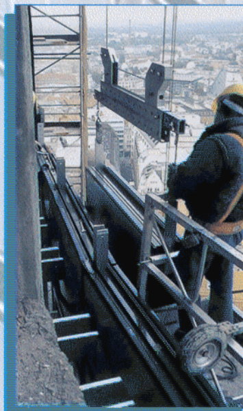
Spreader bar with suspended façade element and an installer on the platform, ready to secure the element.
