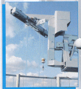
BMU outrigger with integrated material hoist.
