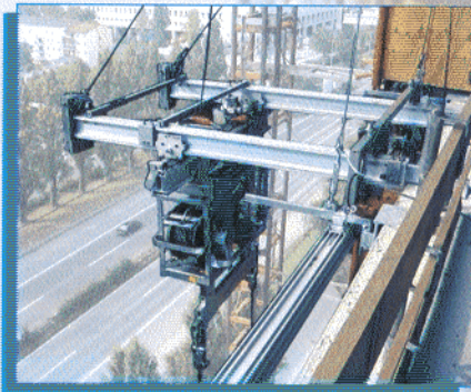
Hoisting unit on the retracted rail section
