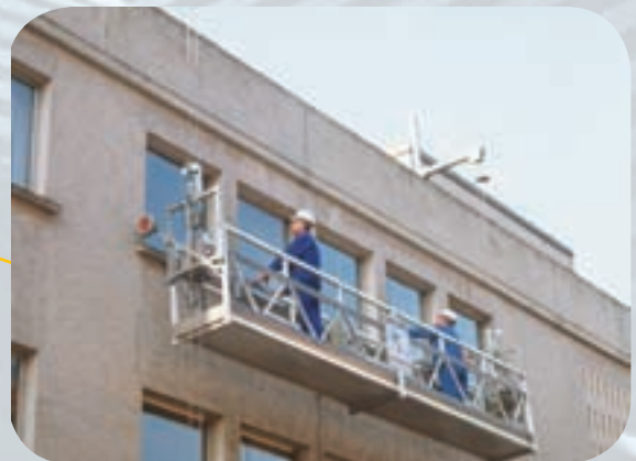
Cradle suspended from Portafix beams
