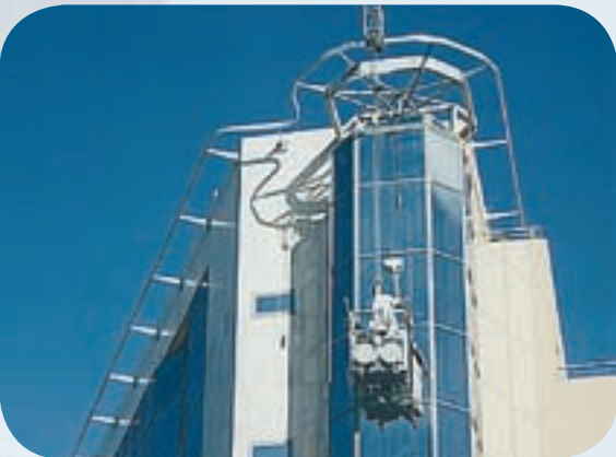
Cradle suspended from trolley traversing on rail
