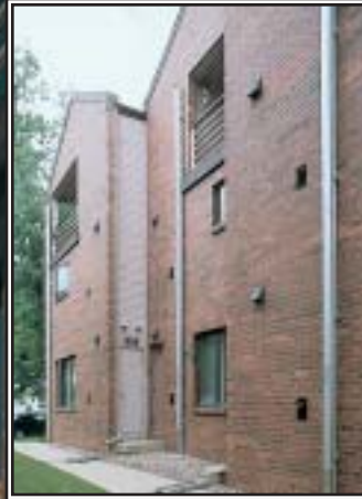
Looks like a drainpipe!
