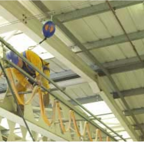
Crane tracks and gentries
