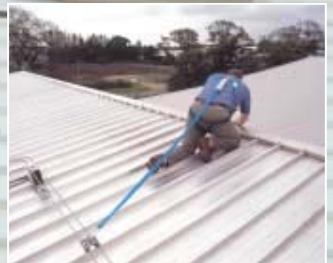
Profile sheet roofs for access and maintenance
